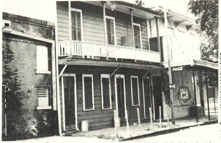
Storyville . . . the last surviving house
